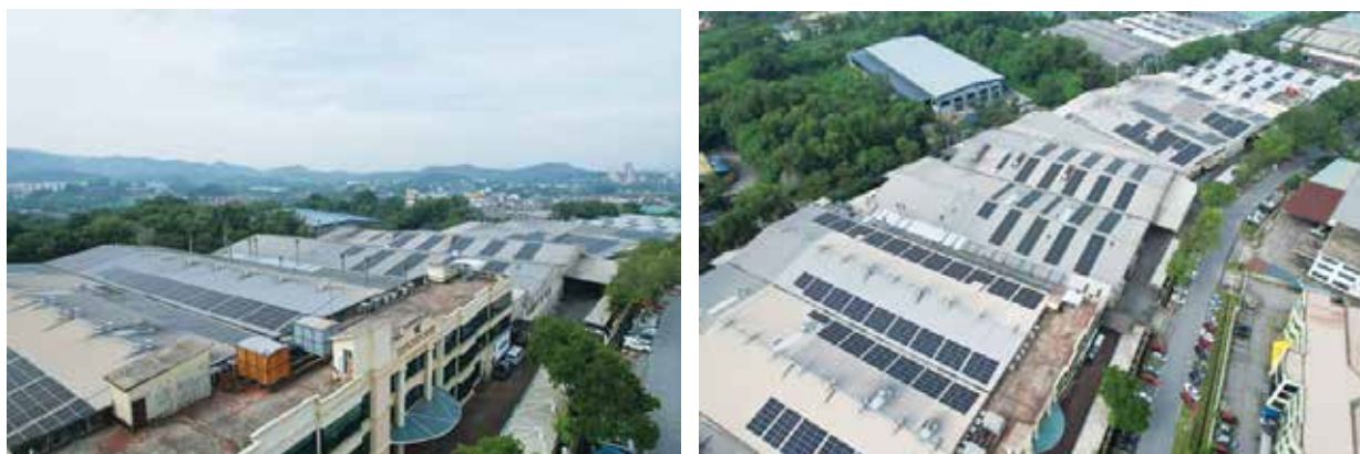
Figure 1 & 2: Installation of solar panels
